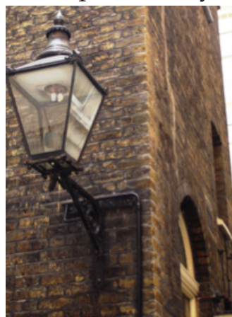
The oldest building in Exchange Court
